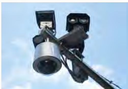
Image NPR (Number Plate Recognition) Capture Camera+Paragon IR Illuminator (Building Entrance)
